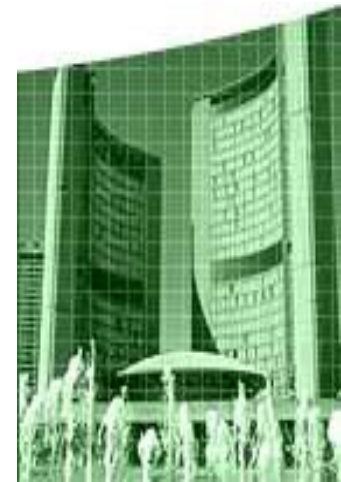
ACCESSING CITY HALL
